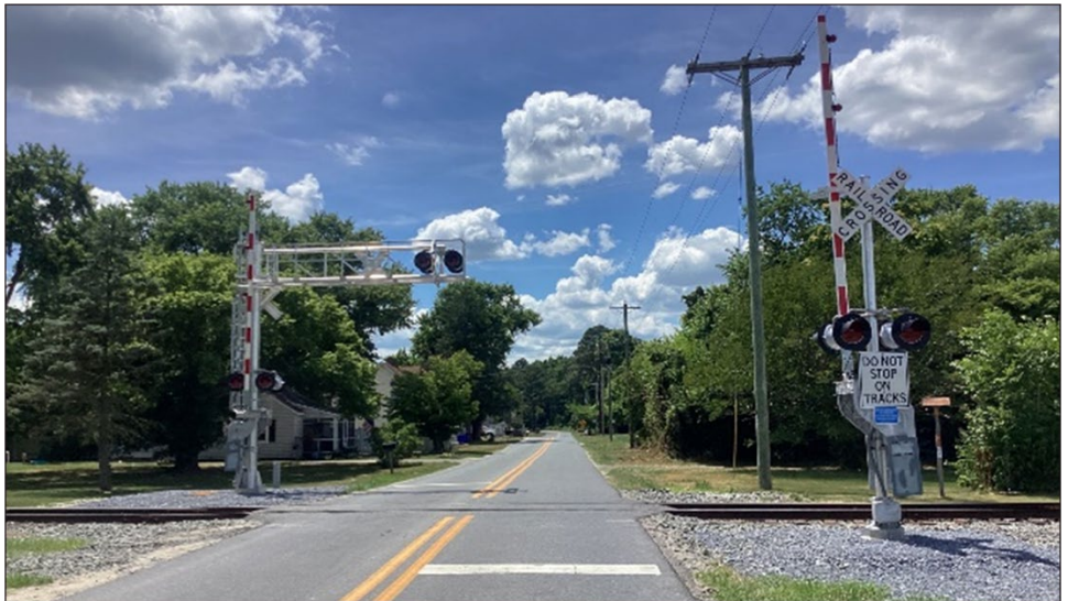
Figure 10: Completed Railway-Highway Crossings Program Project on Bacon's Road in Laurel, Delaware, That Upgraded Signals, Gates, and Lights at a Grade Crossing (#516390T)
