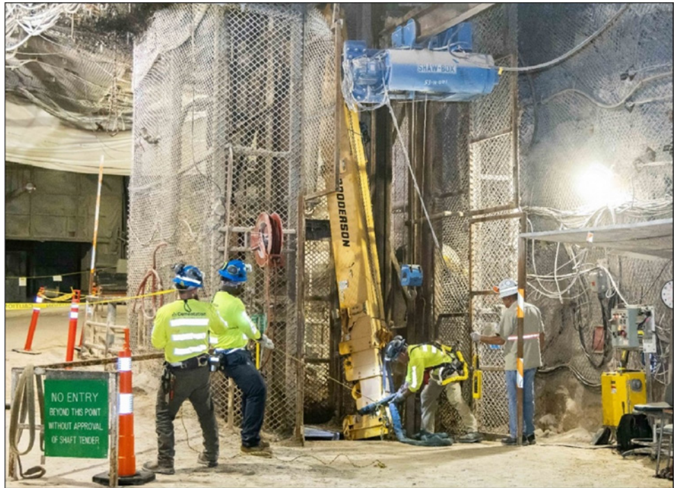
Figure 9: Contractors Refurbishing the Salt Handling Shaft at the Waste Isolation Pilot Plant in New Mexico in 2024
