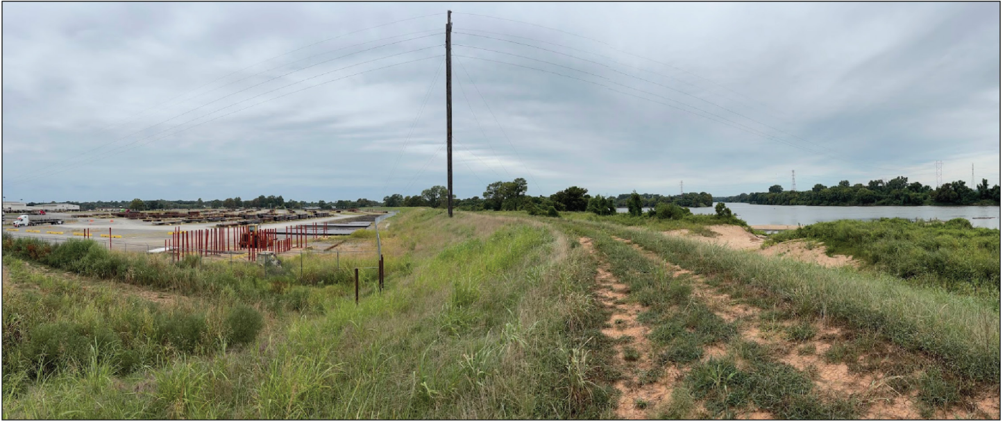
Figure 14: Levee to Protect Inland Port from Flooding in Muskogee, Oklahoma
