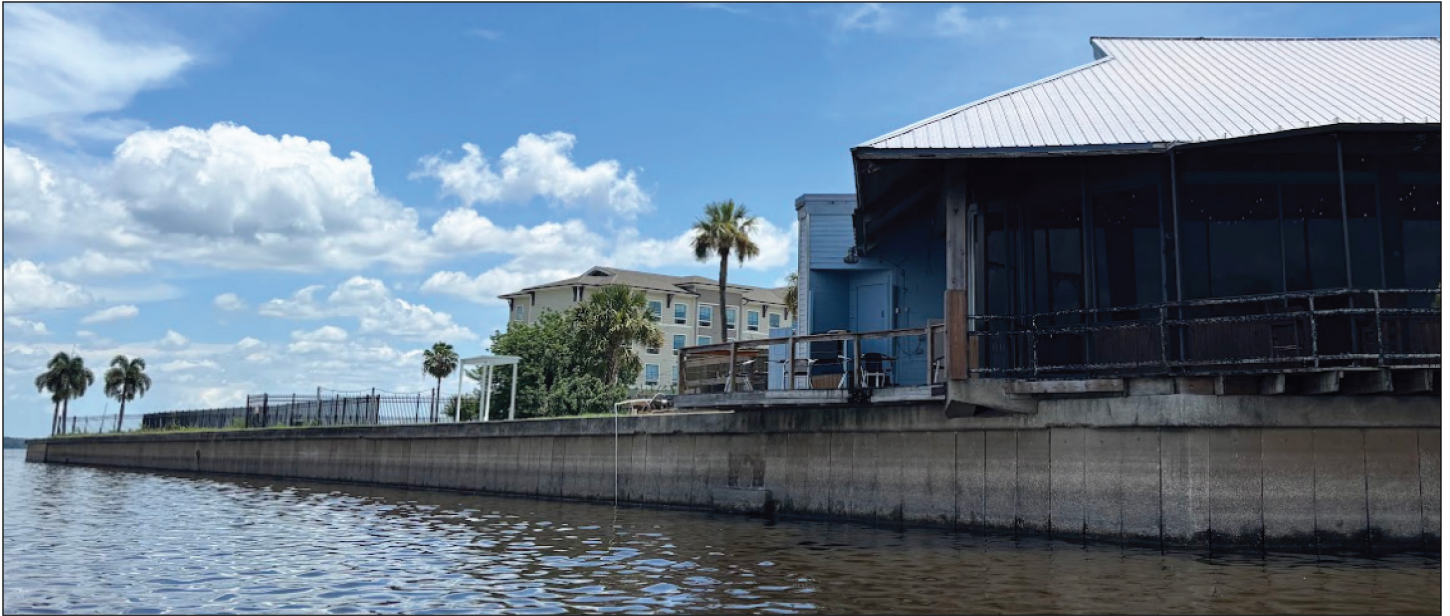
Figure 11: Seawall to Be Elevated Around Marina and Commercial Area in Sanford, Florida
