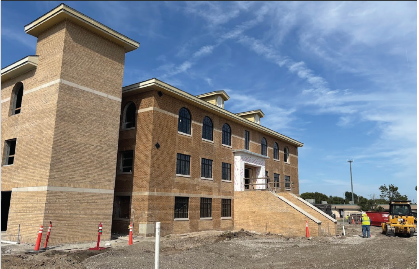
Figure 13: Business Resource Center Under Construction at Former Hospital in Tulsa, Oklahoma
