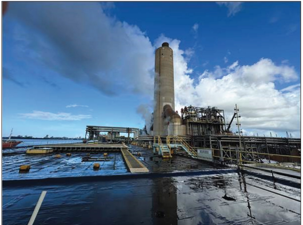
Figure 3: Federal Emergency Management Agency Public Assistance Project Eligible to Receive Community Development Block Grant Funds to Help Cover Cost Share: San Juan Central Generation Station
