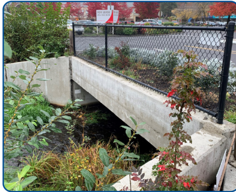
Culvert with a protective headwall that prevents erosion and allows water to pass under a road
