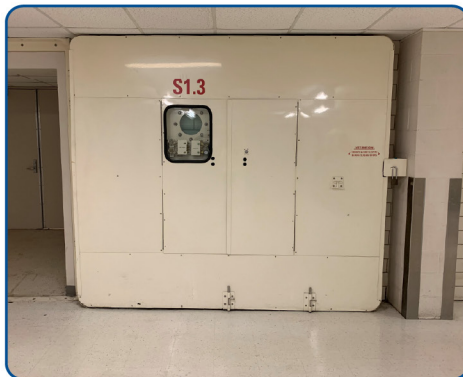
Watertight enclosure to prevent floodwater damage
