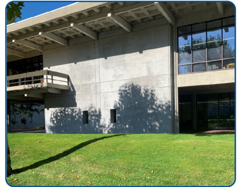
A shear wall that is part of a seismic retrofit of a university library
