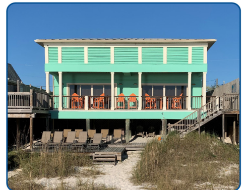
Structure elevation to mitigate flood damage
