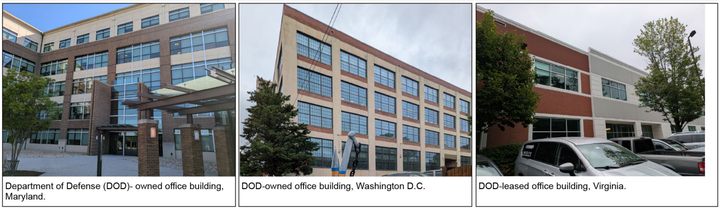
Figure 1: Examples of DOD-Owned and -Leased Office Buildings in the National Capital Region
