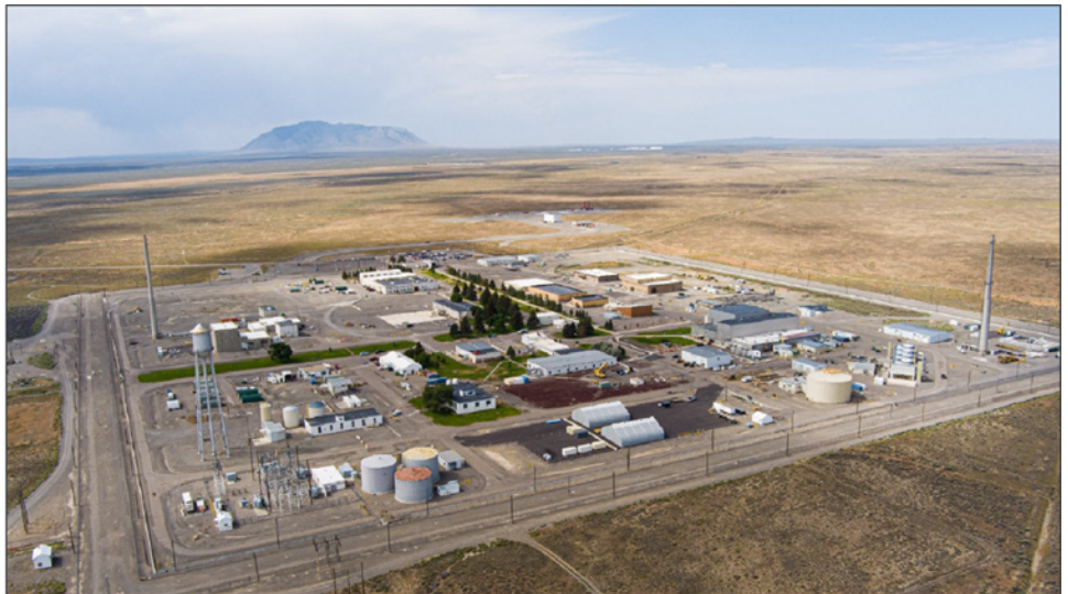
Figure 1: Advanced Test Reactor Complex, Idaho National Laboratory
