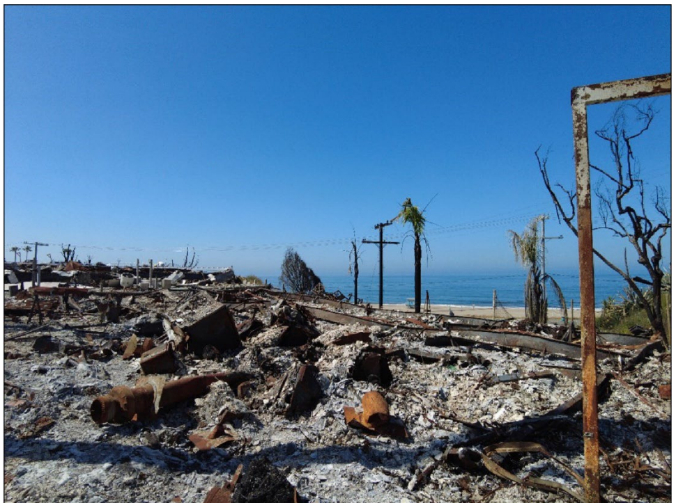
Figure 9: Uncleared Fire Debris at Tahitian Terrace in Pacific Palisades, California, May 2025
