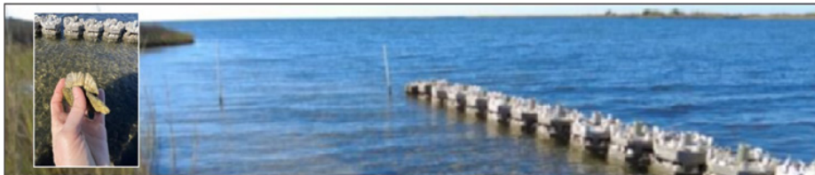
New oyster reefs installed to reduce storm surge damage and slow shoreline erosion. Inset shows young oysters beginning to establish on the reef.
